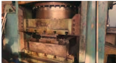
05 Repair of Deformations
